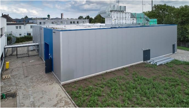
Fig. 5: The completion of the cleanroom building is expected shortly in Q4 2020
